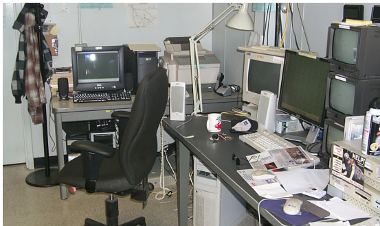
Figure 6. The control room where much of the systems are controlled.
